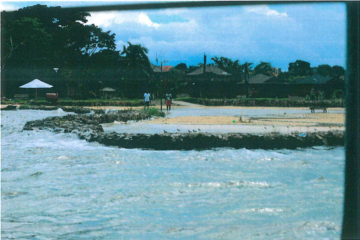
A stretch of hard stones and soil into lake Victoria in Busabala, Wakiso District designed to create more beach space at a resort. The stretch goes as long as 50meters into the lake.Photo taken by Matte on 02/05/2023 for The Environment Shield. Below is an image of remains of a house washed away by water at Mulungu Beach in Munyonyo, kampala.
