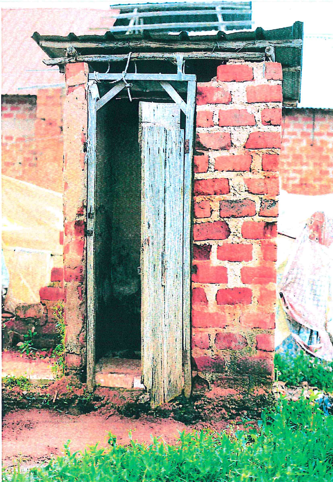
Sanitation in informal settlement in a wetland, human waste mixes with water of the wetland in Kirombe - Butabika - Kampala, Uganda. Documentation done on Tuesday, 9th May, 2023.
